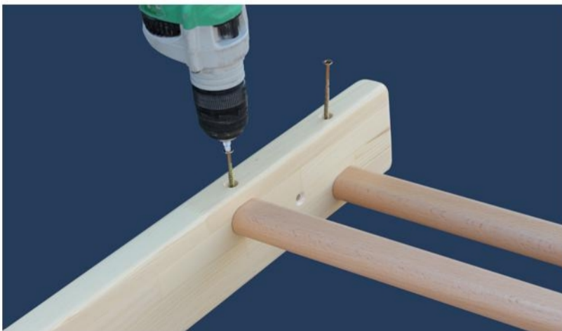
5. Screw the rungs into a place with the short screws.
