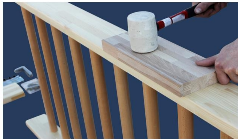
4. Use a wood block and rubber mallet if necessary to fully seat rungs.
