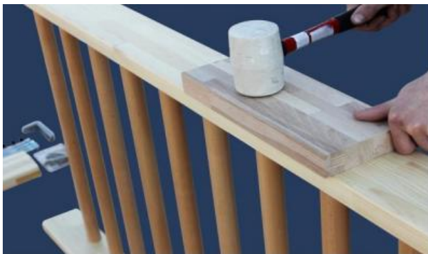
3. Use a wood block and rubber mallet if necessary to fully seat rungs.
